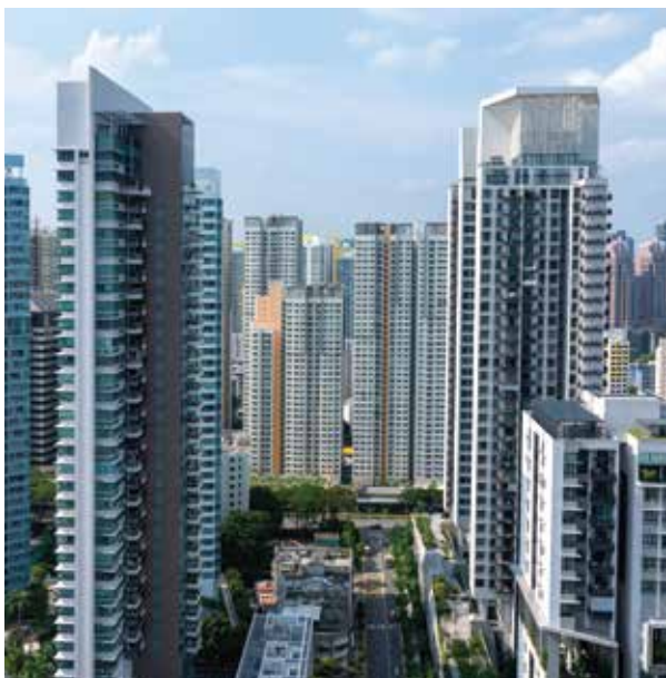
Apartments and High Rise Dwellings.
